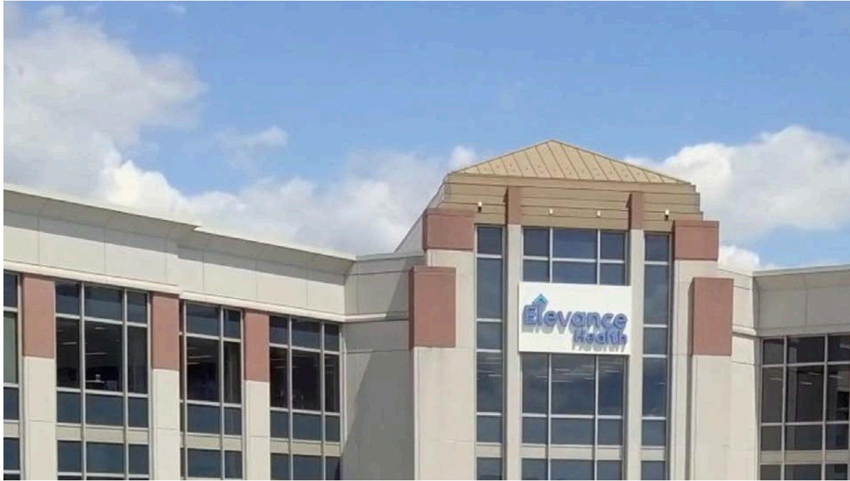
Elevance headquarters in Indianapolis, Indiana. Permission granted by Elevance Health.
